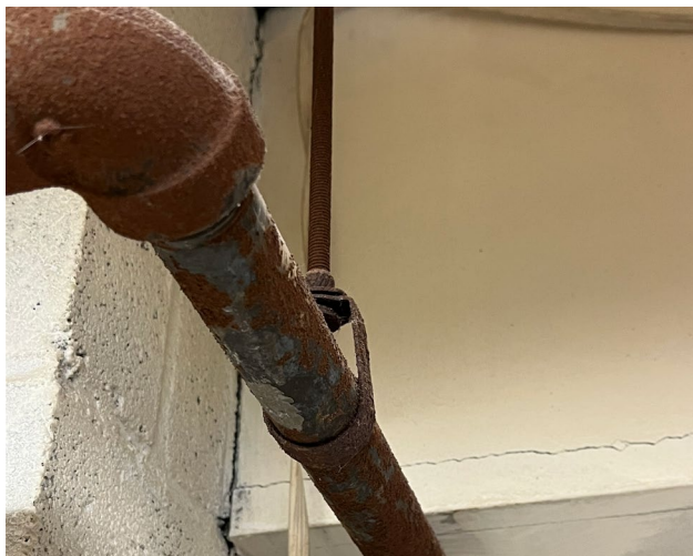
Visible plumbing before sanding.
