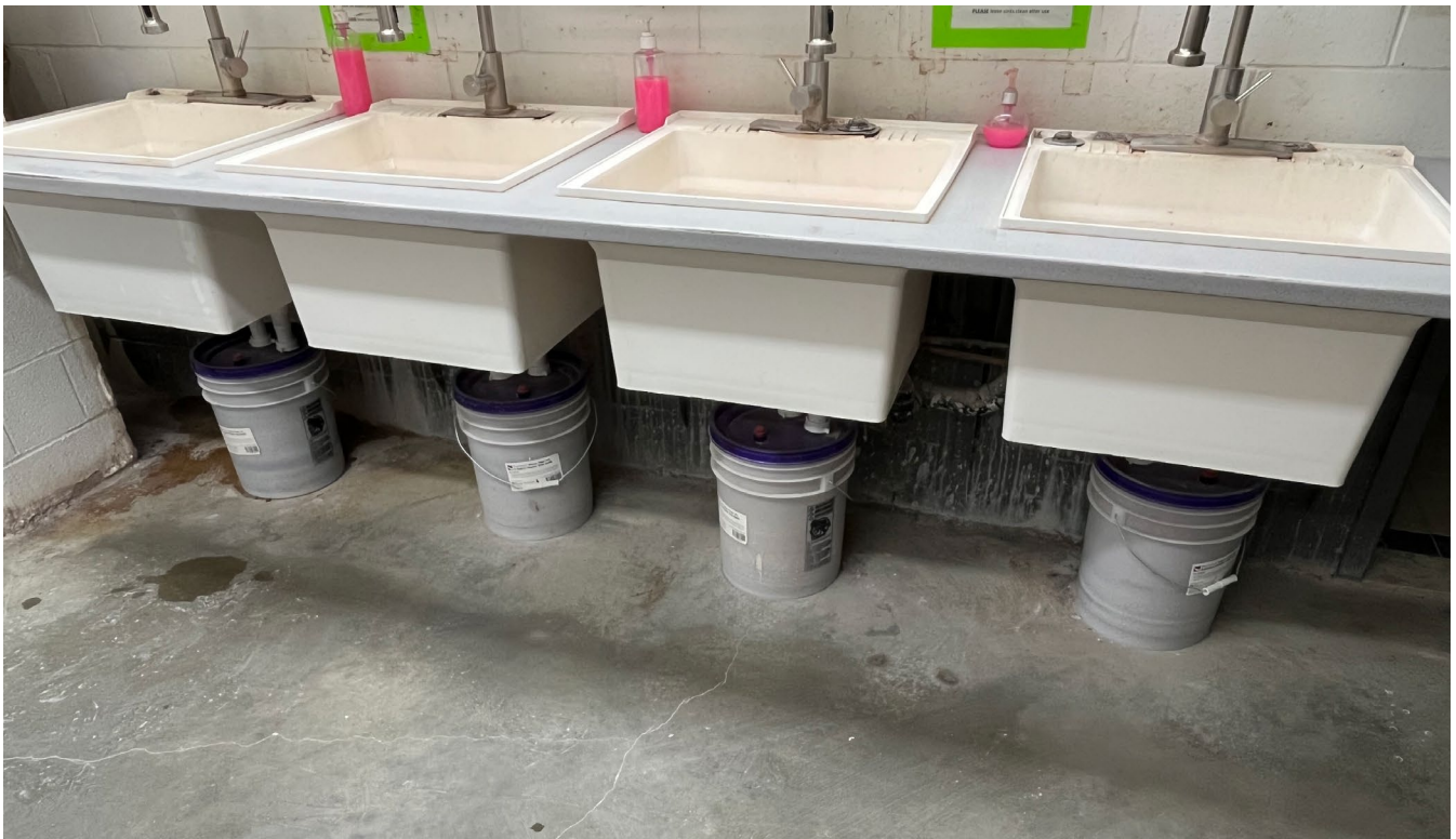
New clay traps, under the sinks in the ceramics studio.
