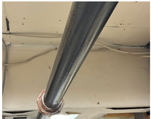
Visible plumbing after sanding.
